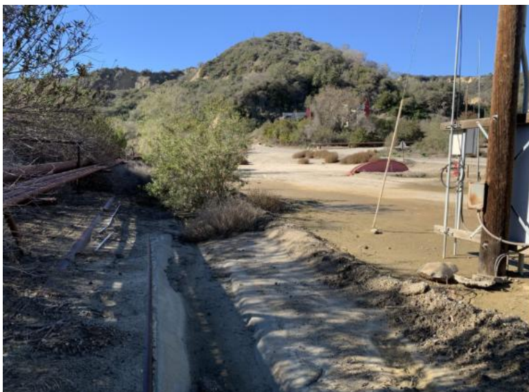
Exhibit 2-24: Existing stormwater swale at the Devil’s Canyon Road Site
