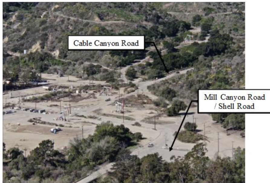
Exhibit 2-13: West-facing view of the north side of the existing Devil’s Canyon Road Site, Mill Canyon Road/Shell Road, and Cable Canyon Road
