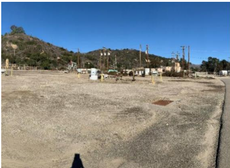
Exhibit 2-23: Existing stormwater drain at the Devil’s Canyon Road Site
