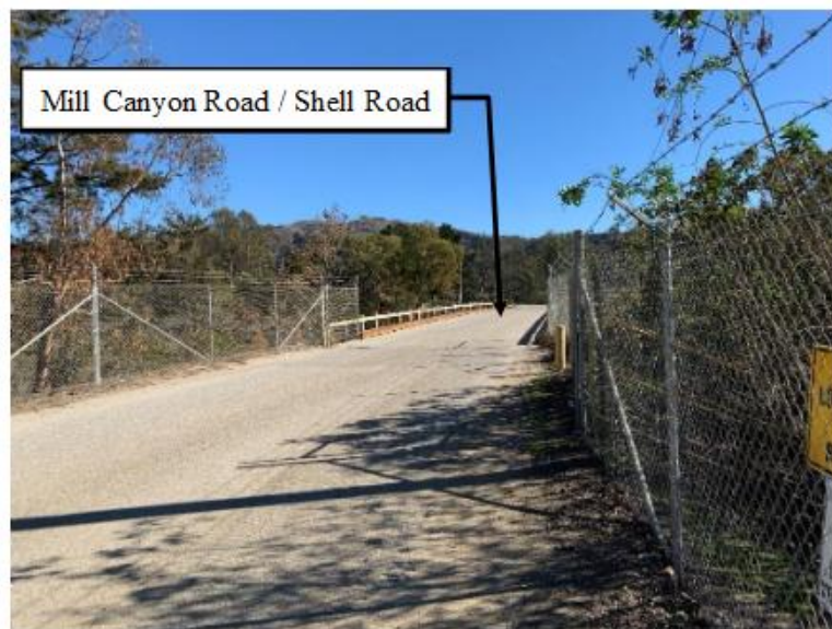
Exhibit 2-2: East-facing view of the west side of the bridge crossing the Ventura River to access the Devil's Canyon Road Site
