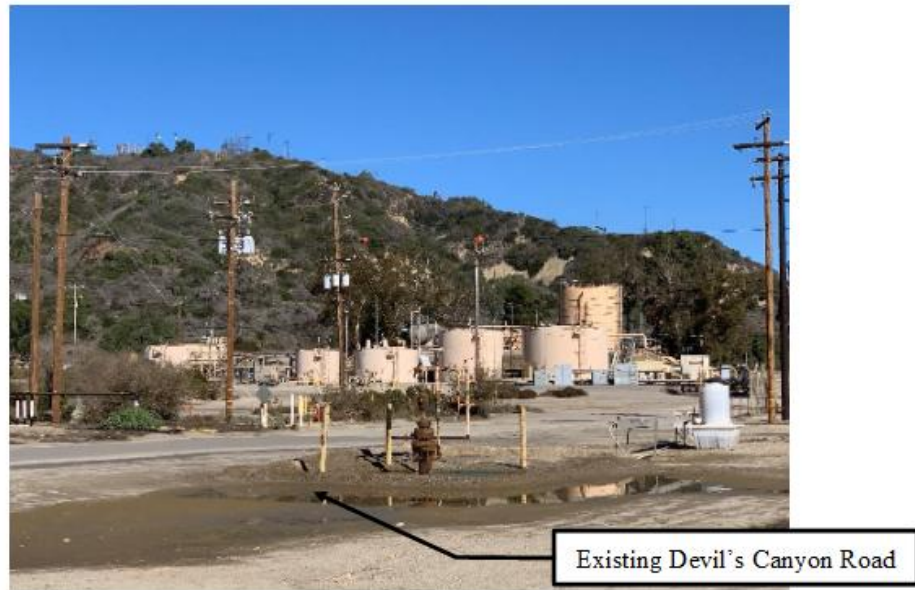
Exhibit 2-7: Existing conditions at the Devil's Canyon Road Site (Close-Up of Tanks)
