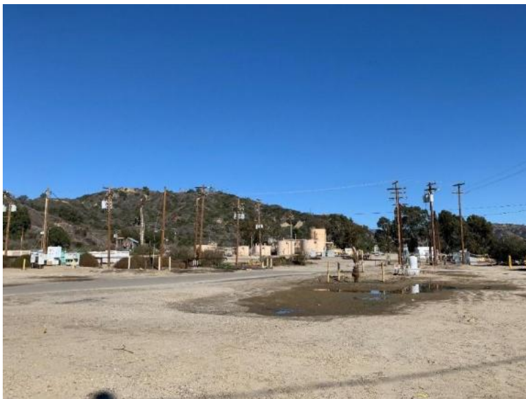
Exhibit 2-14: Existing conditions and oil facility at the Devil's Canyon Road Site
